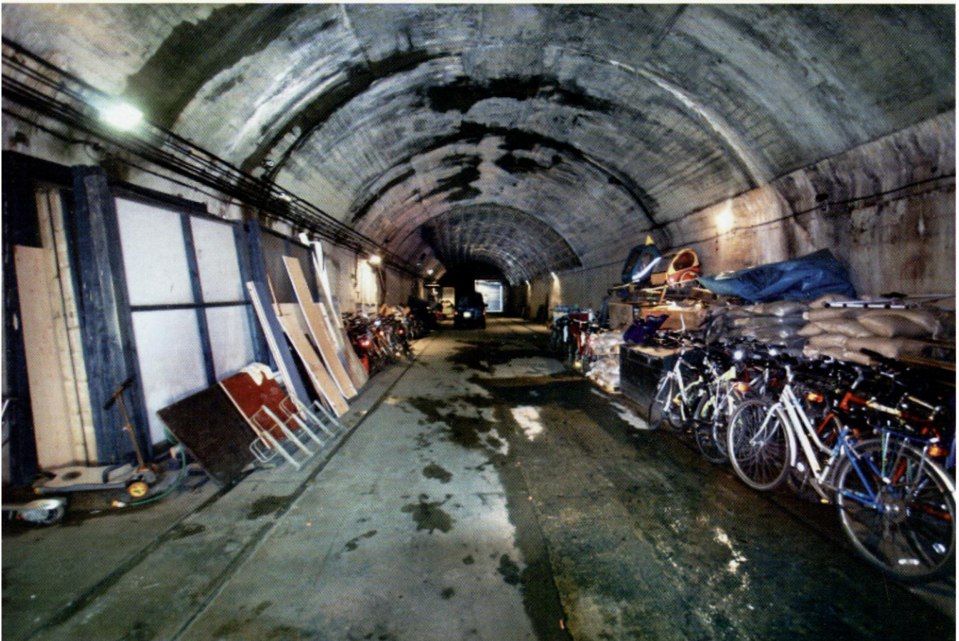
Just inside the entrance portal to the 1898 railway tunnel at St Aubin, later adapted by the Germans as Ho5. The tunnel, part of which is now a depot for bicycle hire, was converted to metre gauge by the occupiers - a section of this track is visible on the right. 60 cm-gauge track is seen on the left; this was laid into the new side storage tunnels. Photo Nick Catford
